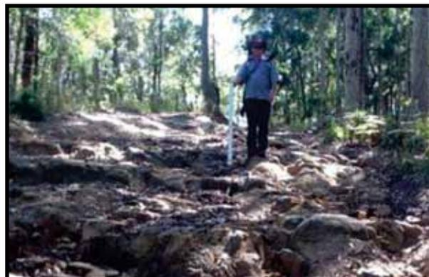
*(Low range 4WD necessary, not suitable for use as a fire trail. Requires reconstruction. Trail may be completely impassable in places.)*
