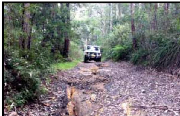
*(May still be usable but major works are required. Insufficient surface material, non existent drainage, inadequate crossfall etc. Low range 4WD necessary in places.)*
